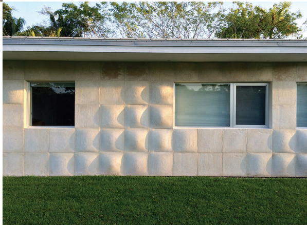
Shadows cast in the morning sunlight on the south facade.
