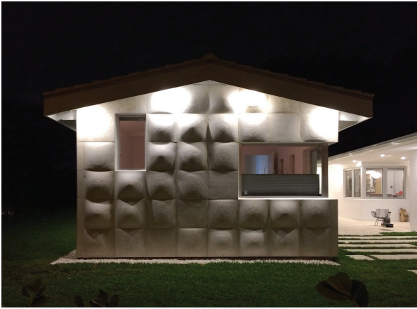
Front facade of house, showing location of windows within the grid of exterior wall panels.
