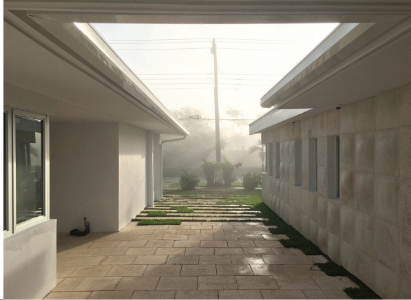
View of courtyard, where the textured panels contrast with the existing smooth walls of the storage room.
